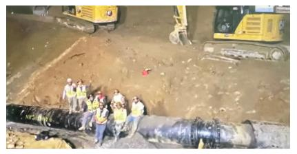
In the early hours of this morning, around 1:30 AM, T&K Utilities connected North Folk's 36-inch bypass line to the water distribution system. What a monumental time for Asheville! There's still a lot of work to do before customers will start receiving water, but that work is being done, and
